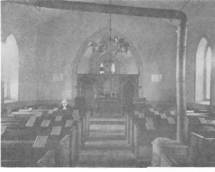
Interior of Old Salem Church Before Restoration
